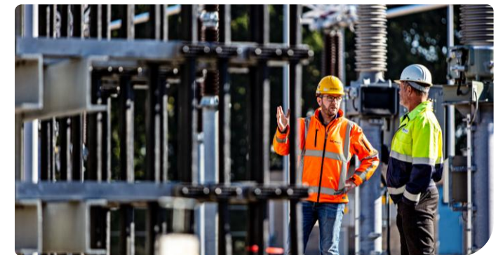
Maasbracht high-voltage substation extension
